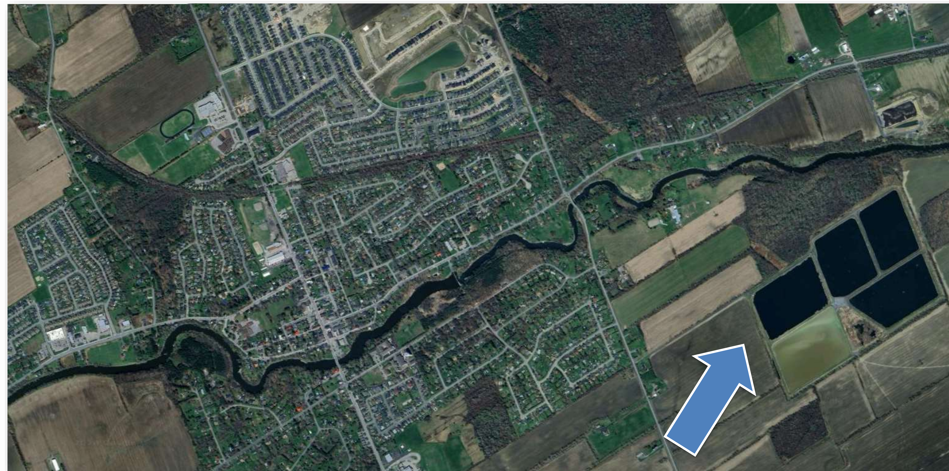
Russell Wastewater Treatment Plant
