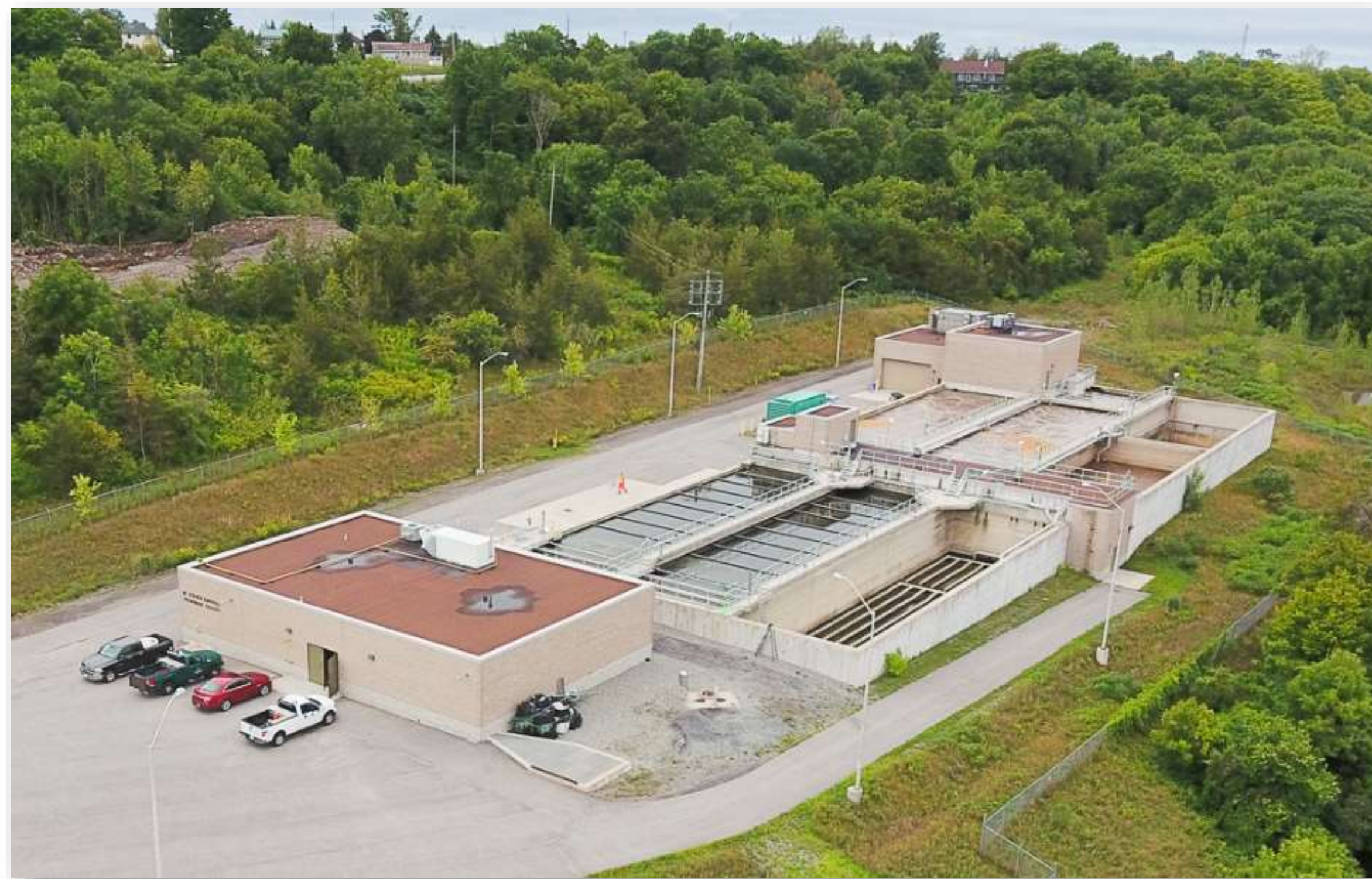
Mechanical Wastewater Treatment Plant
