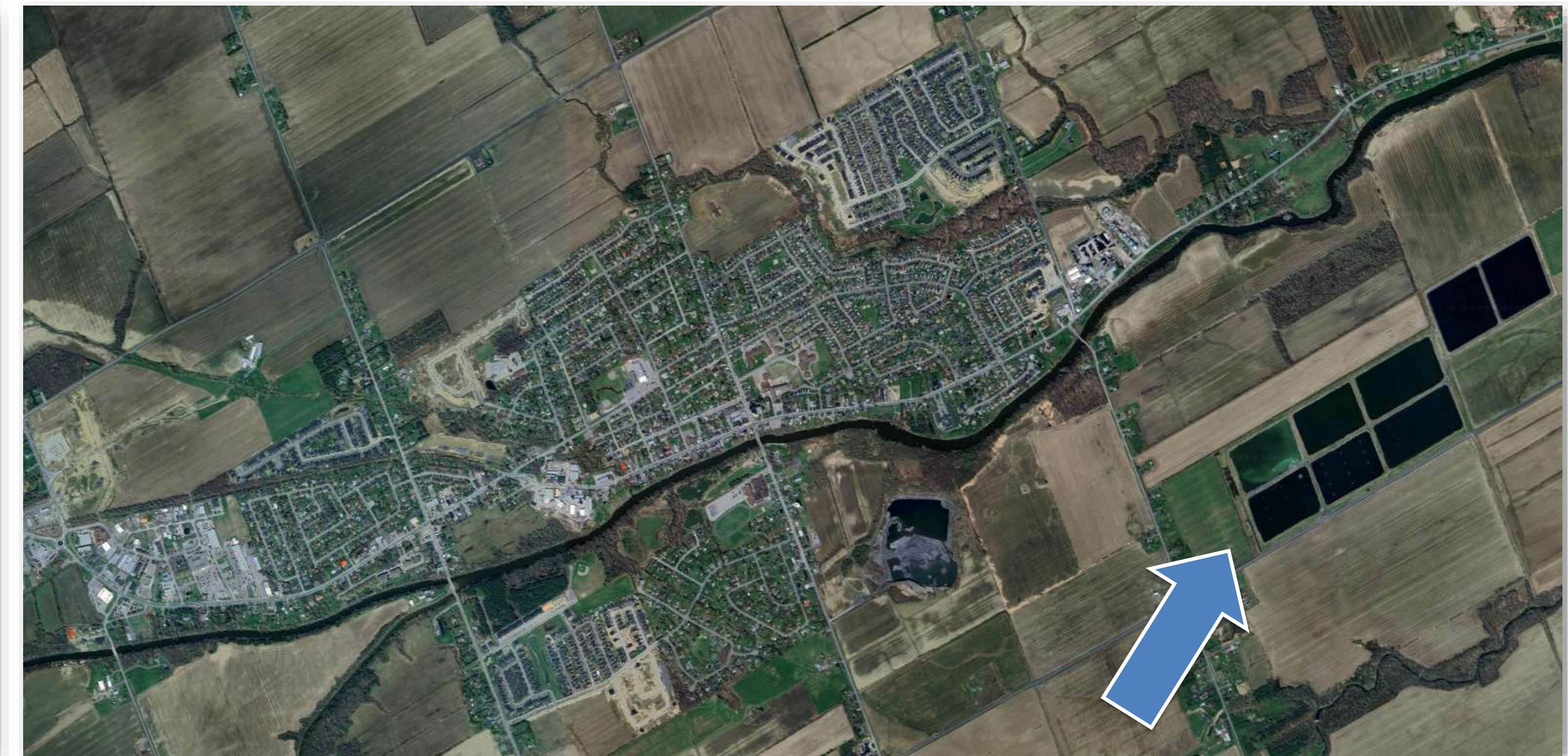
Embrun Wastewater Treatment Plant
