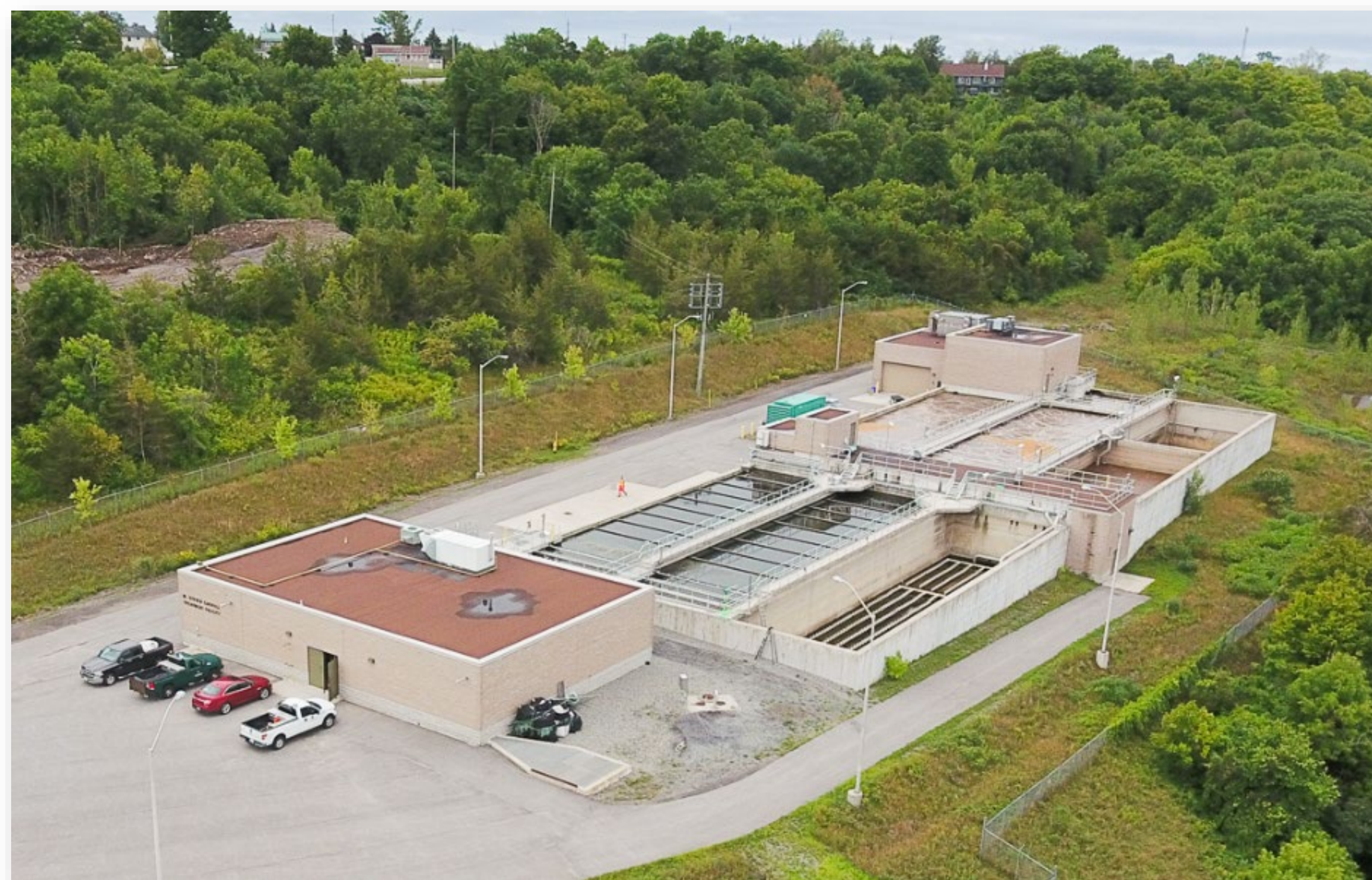
Mechanical Wastewater Treatment Plant
