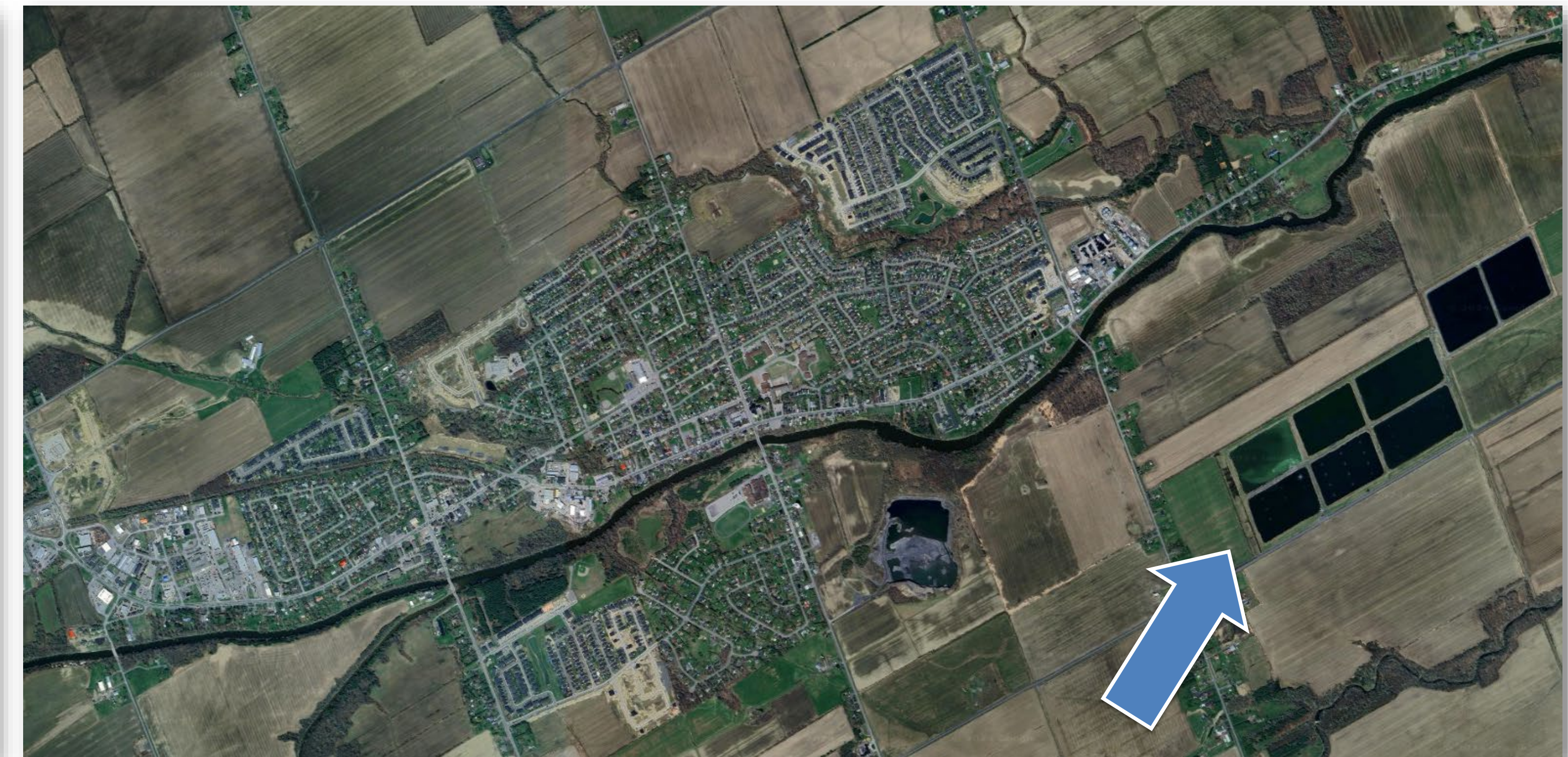
Embrun Wastewater Treatment Plant
