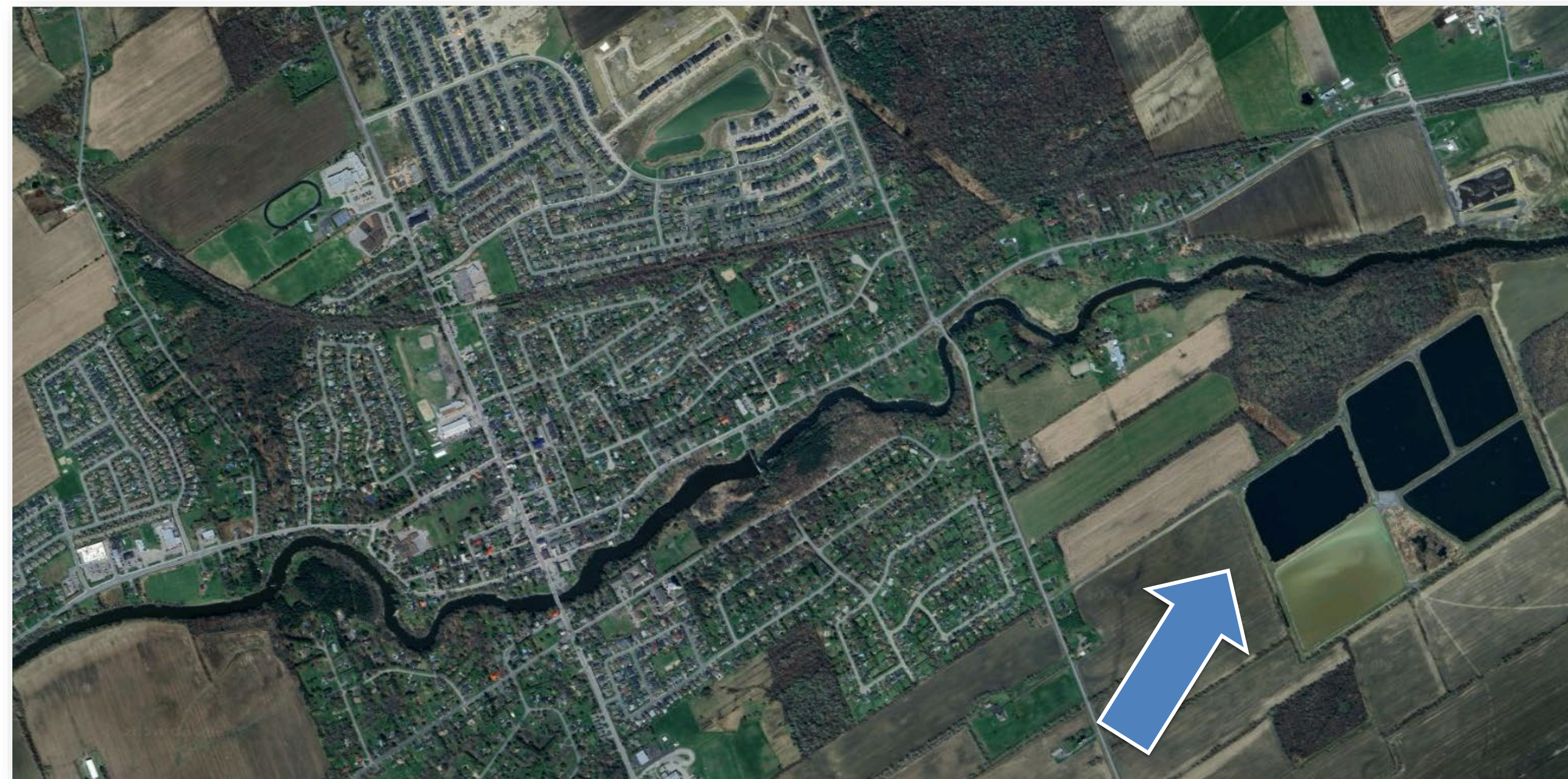
Russell Wastewater Treatment Plant
